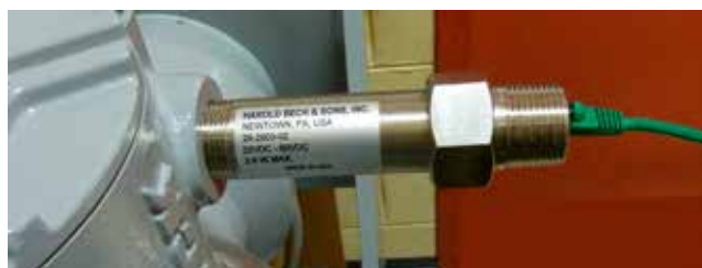
INSTALLED BECK MODBUS TCP ADAPTER
