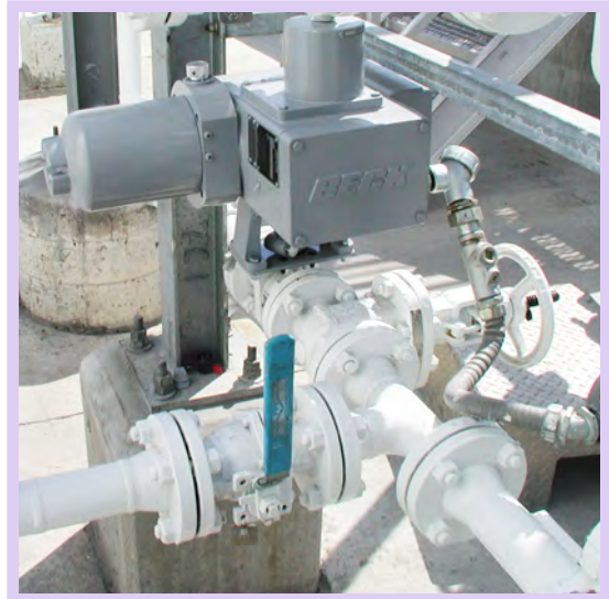
Figure 1 Beck IIE-169 Rotary Valve Actuator on Ethanol/Gasoline Blending Application. [Hazardous Location Rated Class I Div 2]
