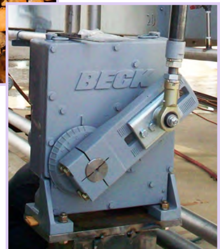
Figure 1 ID Fan Damper - Beck Electric Actuator
