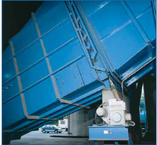
Beck actuator installed on a parallel blade inlet damper.
