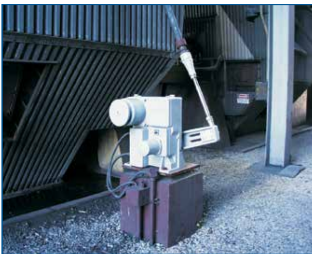
Beck Group 22 actuator installed on a damper.
